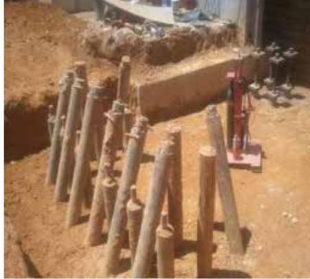
some very challenging karst ground conditions, with limestone rock formations and which have been prone to sink holes. Micropiles ranged in size from 9-5/8", 7", and 5-1/2" diameter steel casing, reinforced with a full length #18, #20 or #24 Grade 75 Nucor Skyline threaded bar. This micropile foundation design allowed for the building and structural loads to be transferred to more competent rock formations deep underground. Additionally, these same difficult sub-surface ground
